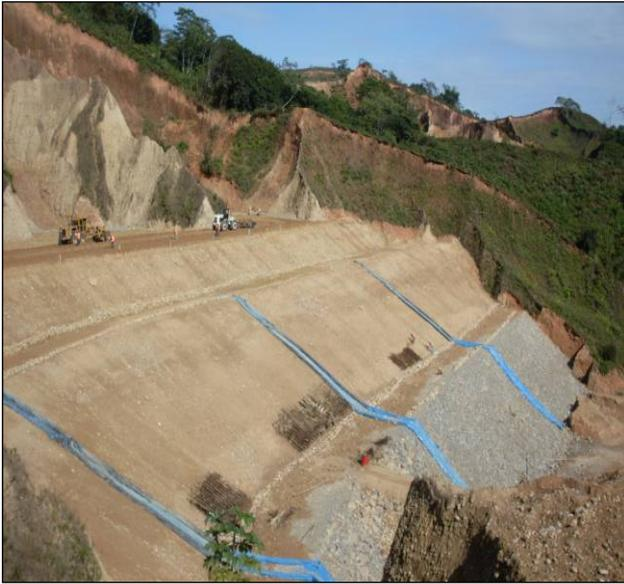
Figure 4. Conformation of embankments
