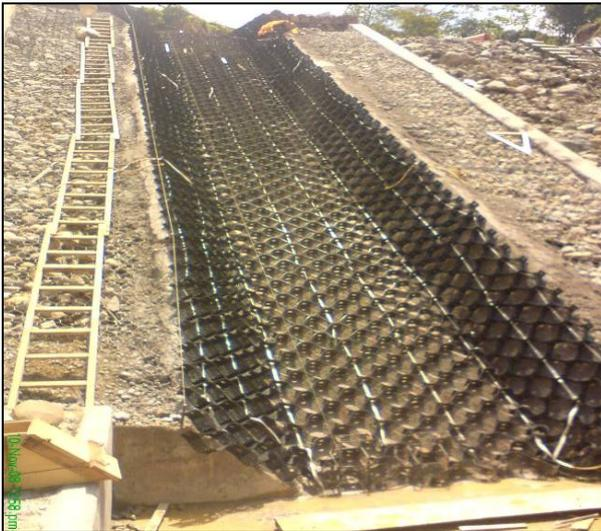
Figure 6. Installation of the geo-cellular confinement system in fast.
