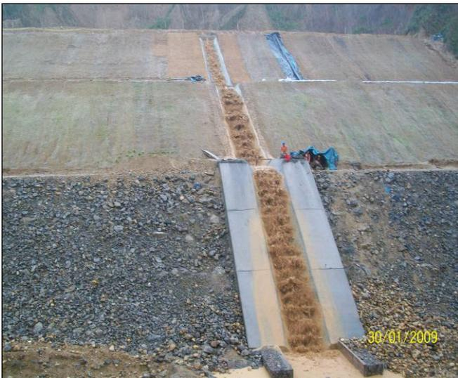
Figure 10. Energy absorbers working during construction (2)
