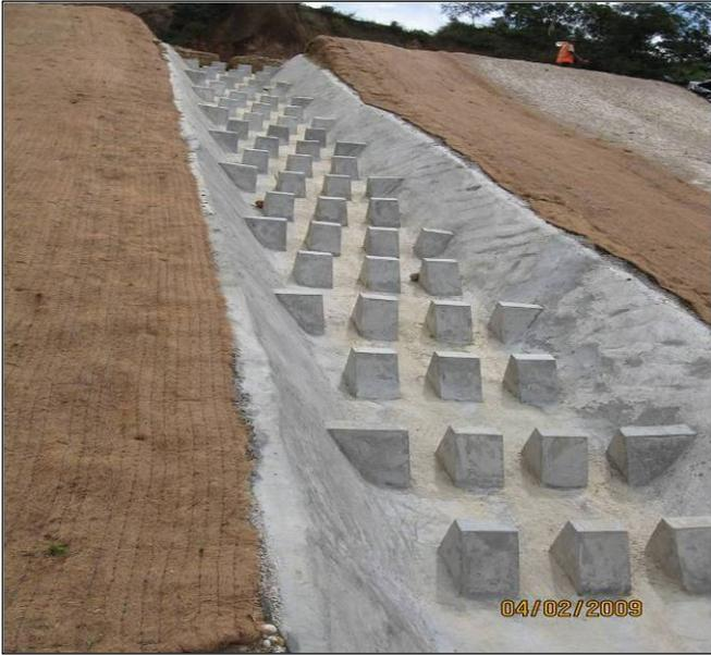
Figure 8. Hydraulic energy absorbers
