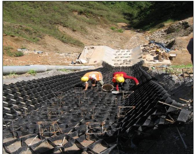
Figure 7. Installation of energy dissipaters
