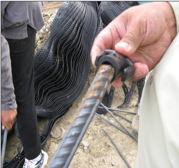
Figure 2. Clip ATRA and corrugate iron stakes.
